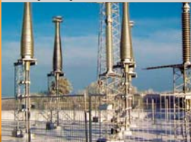
Underground High-Voltage and Extra-High-Voltage Cable
