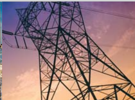
Bare Overhead High-Voltage Transmission and Distribution Cables
